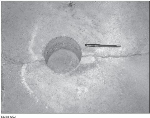
Figure 3: Example of Floor Cracks in the KMCC
