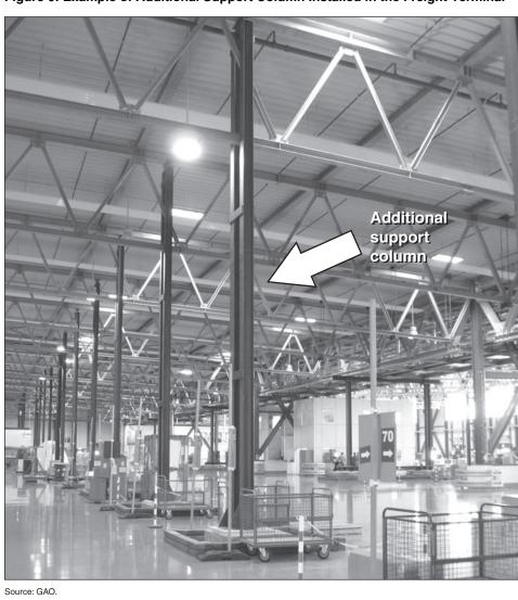
Figure 6: Example of Additional Support Column Installed in the Freight Terminal
